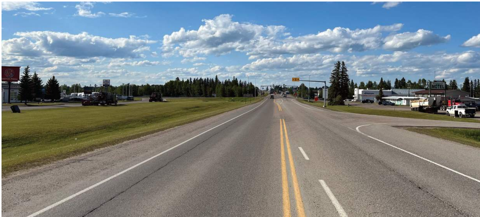
Highway 11 Looking North towards 42 Avenue
