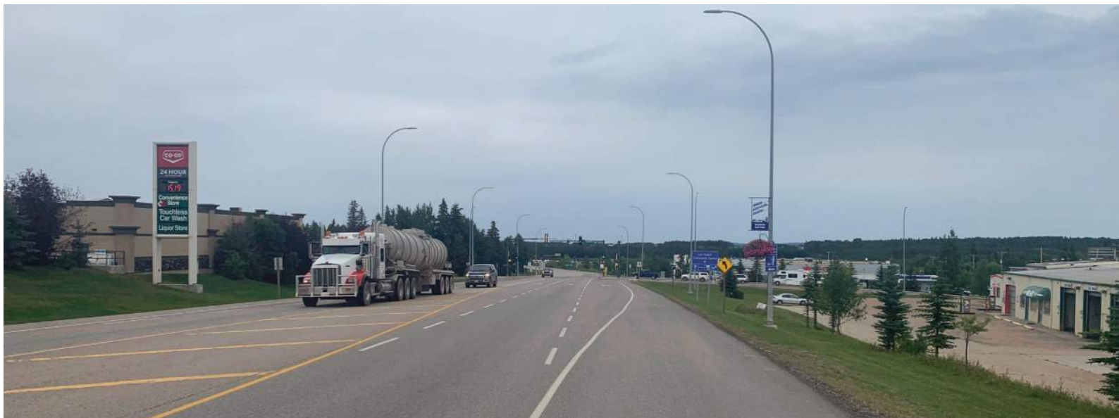
Highway 11 Looking North towards 53 Avenue
