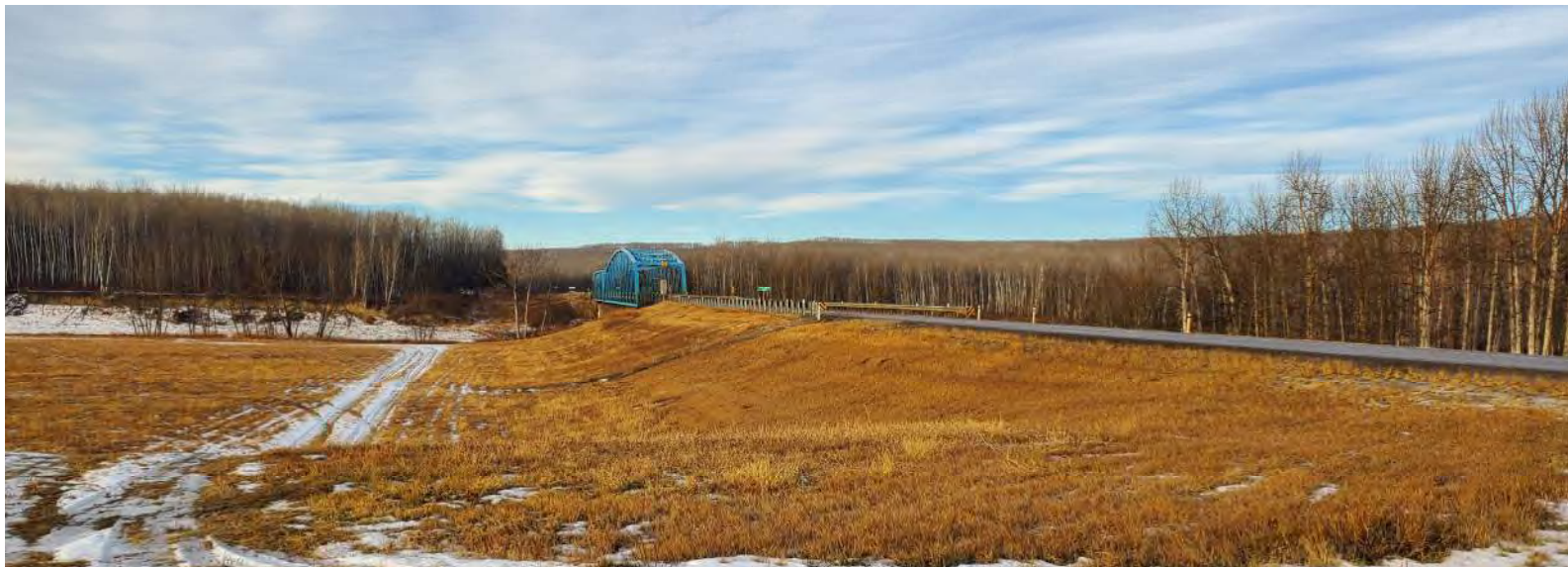
Highway 744 Looking Northwest Across the Little Smoky River Valley
