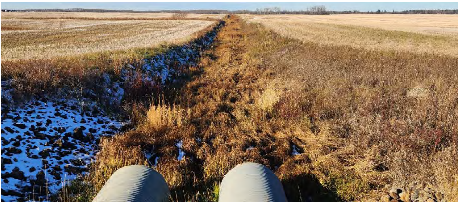
Peavine Erosion Control Channel, Looking West
