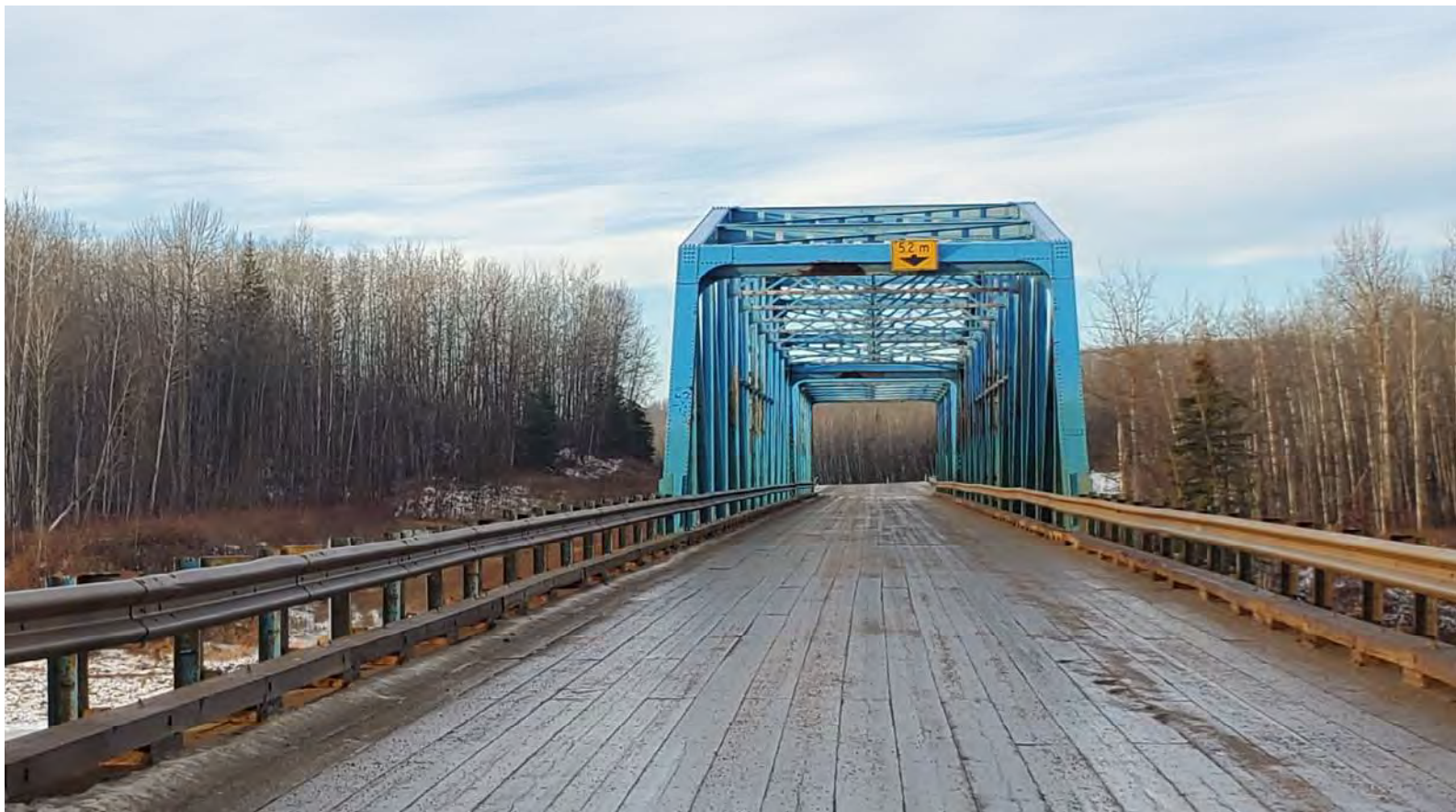
Highway 744, Looking West Across the Little Smoky River Valley
