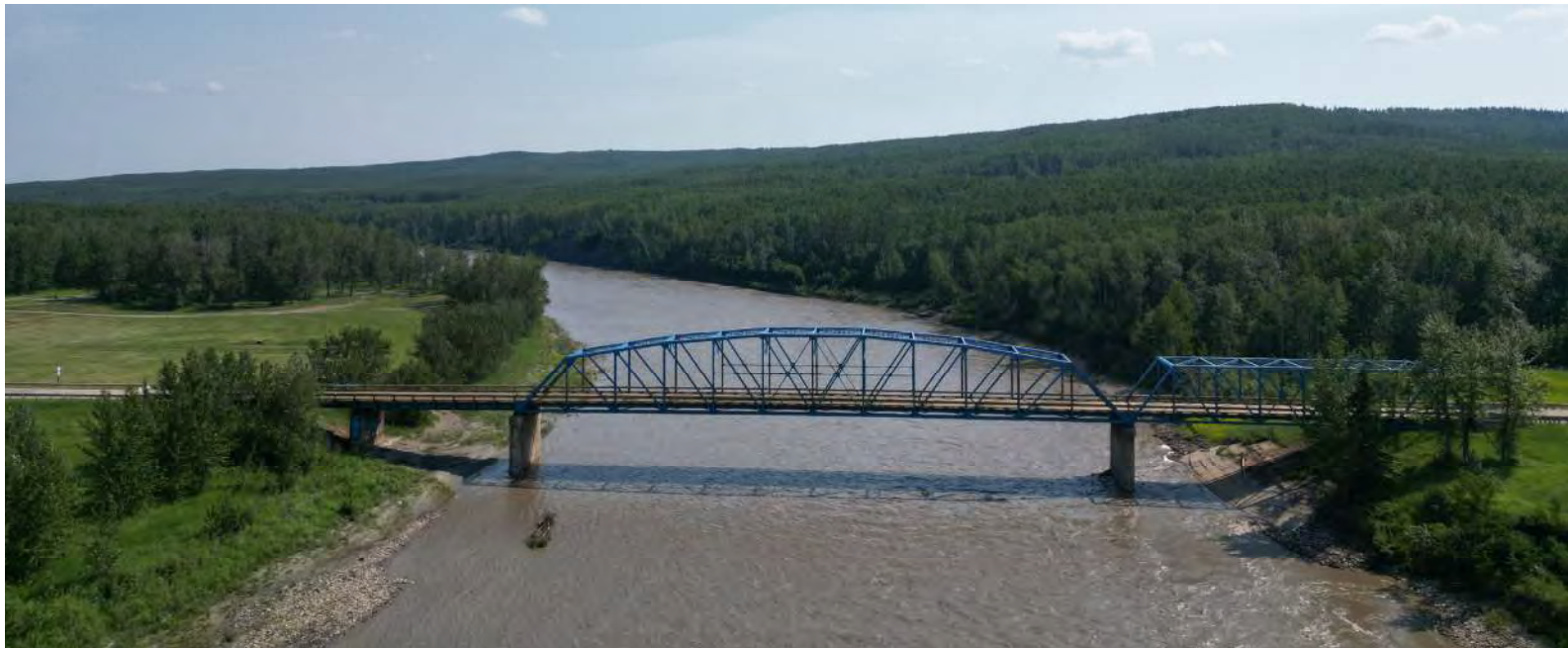
Highway 744 Smoky River Bridge Looking South
