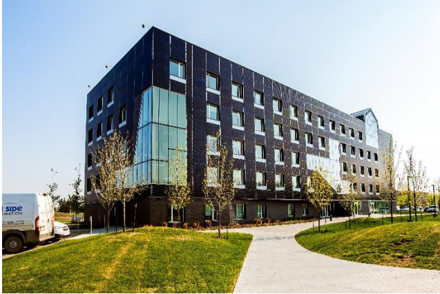
Fig. 1: Red Deer Polytechnic Student Residence with black BIPV wall panels (used with permission by Clark Builders , photographed by Crystal Puim Photography)
